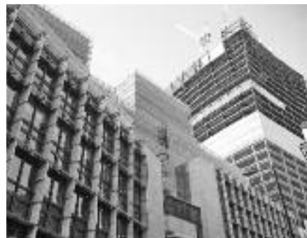
Plantation Place by Arup e nuovo cantiere 2012
